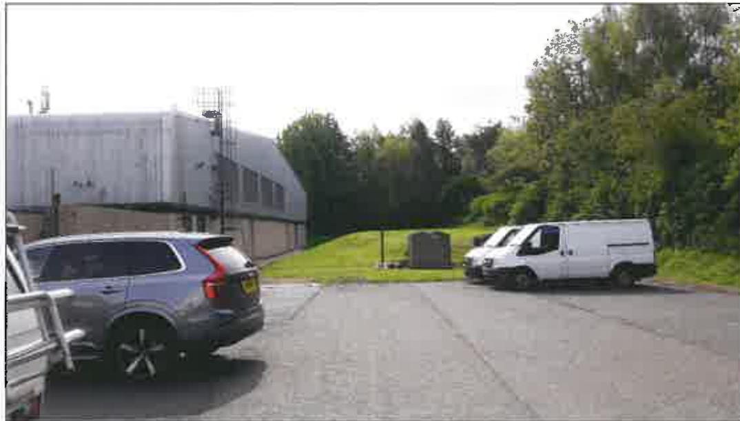
Fig 2: Existing Car parking and south west elevation
