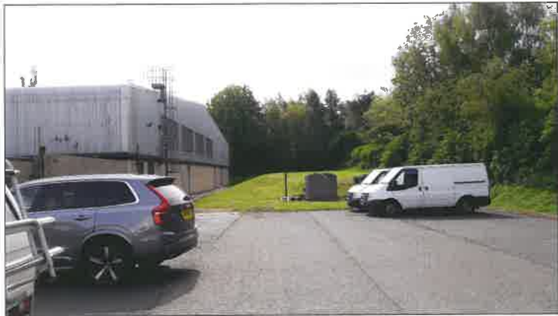
Fig 2: Existing Car parking and south west elevation
